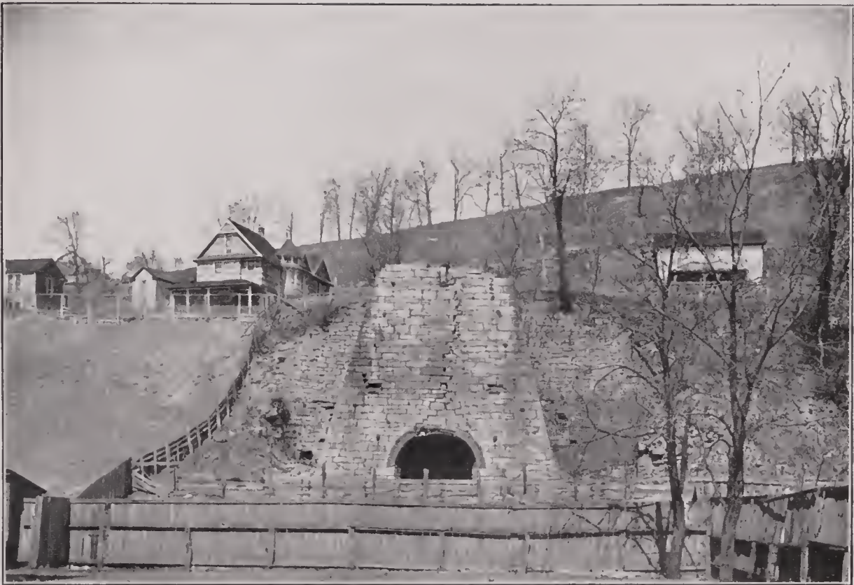
FIG. 1.—RUIN OF BLAST FURNACE, LONACONING, ALLEGANY COUNTY.
